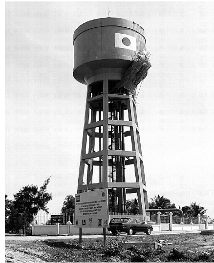
Photo-1 Constructed Water Tank
